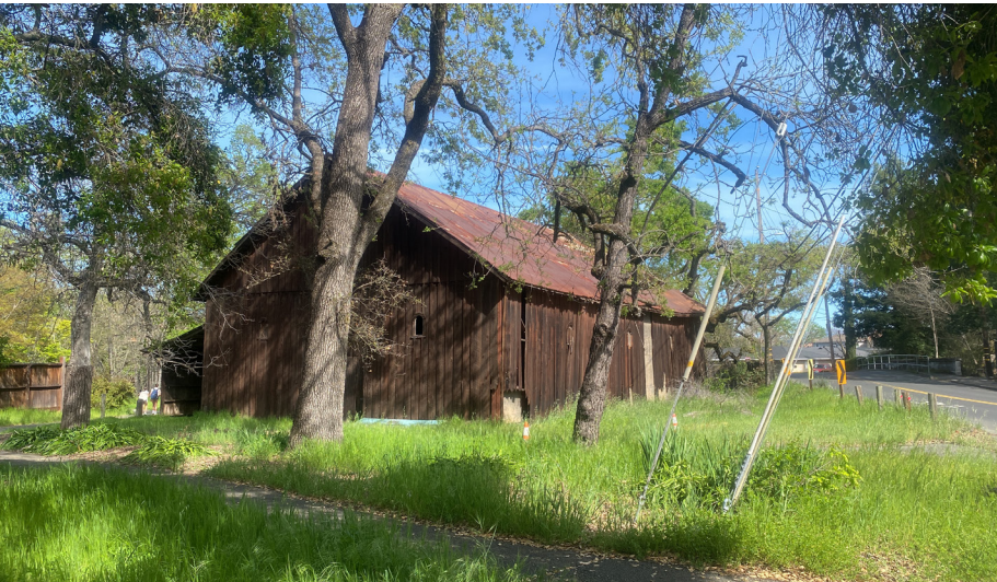
Existing conditions at Signorelli Barn,
