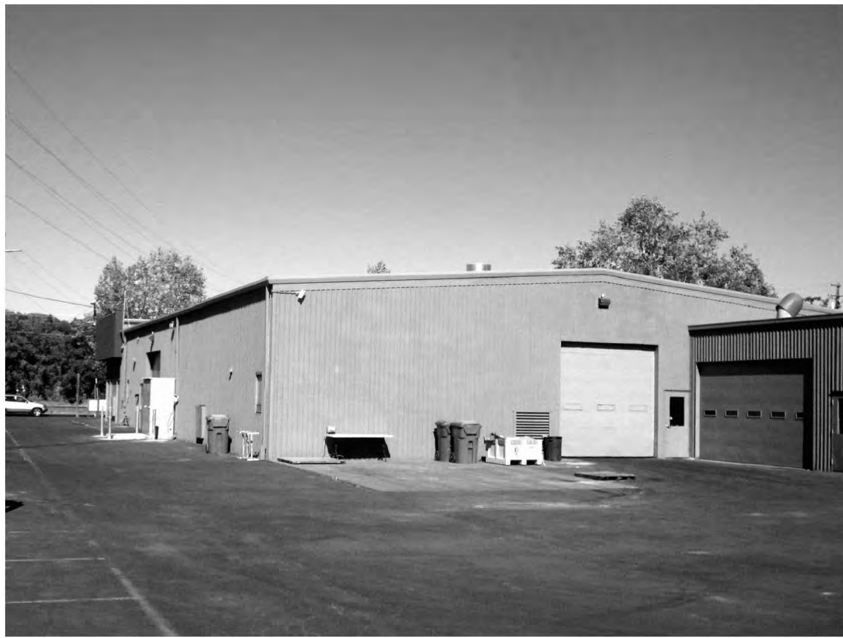
4 VIEW OF BACK OF EXISTING WINERY SCALE: NONE
