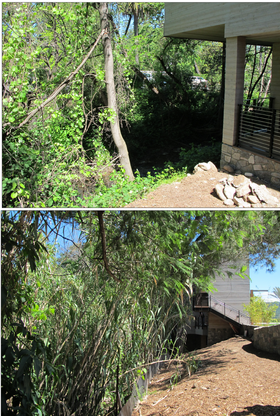
Existing Conditions Las Alcobas Bridge St. Helena, California
