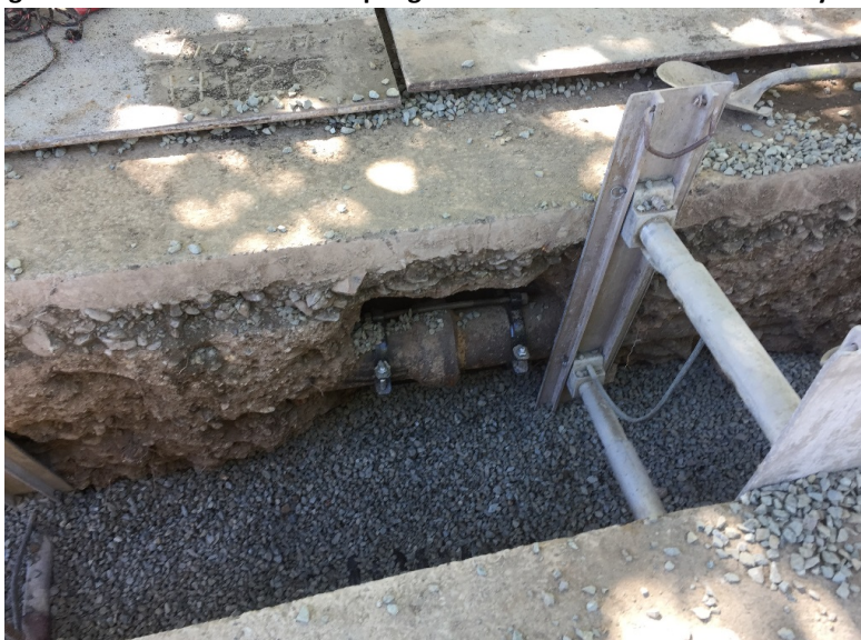
Some of the many Water and Gas Service Crossing the Trench
