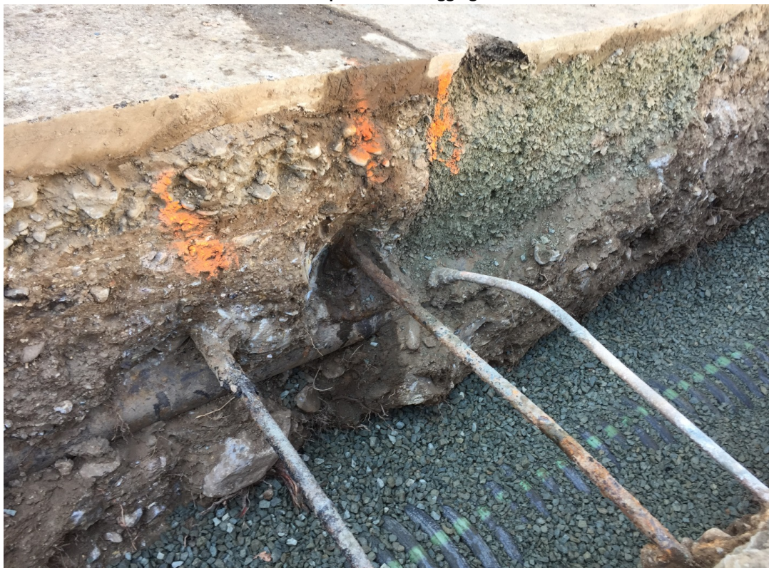
Section Illustrating Storm Drains Close Proximally to Water Main and Service Connections which Required Hand Digging
