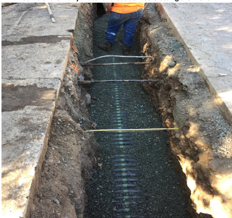
Some of the many Water and Gas Service Crossing the Trench
