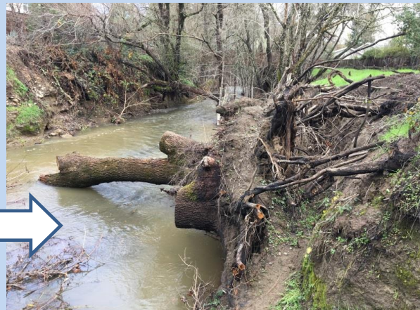
Photo 2. Downed tree limbed, left in place, and modified slightly to function as a weir.
