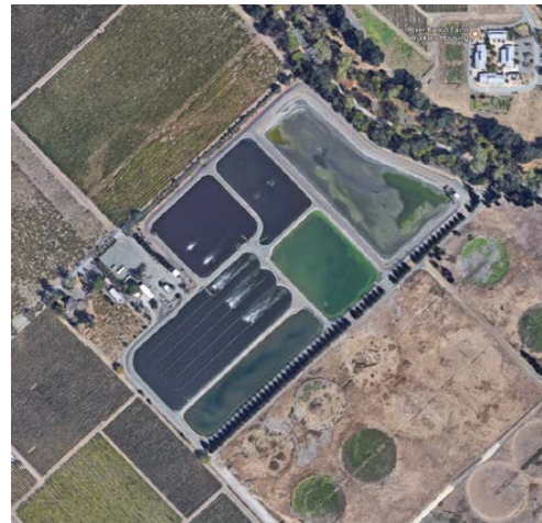
Figure 4.1 Wastewater Treatment Plant Phase I Upgrades. Estimated project cost of $8,430,514.
