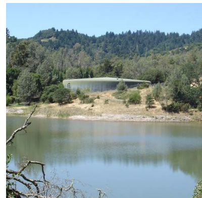
Figure 1.2 Tank 2 Rehabilitation. Estimated project cost of $750,000
