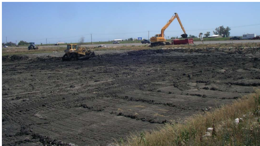
Figure 24 – Rototiller and Long Reach Excavator at Maxwell WWTP Pond
