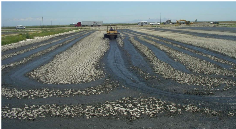
Figure 23 – Rototiller Mixing and Drying Sludge at Maxwell WWTP Pond
