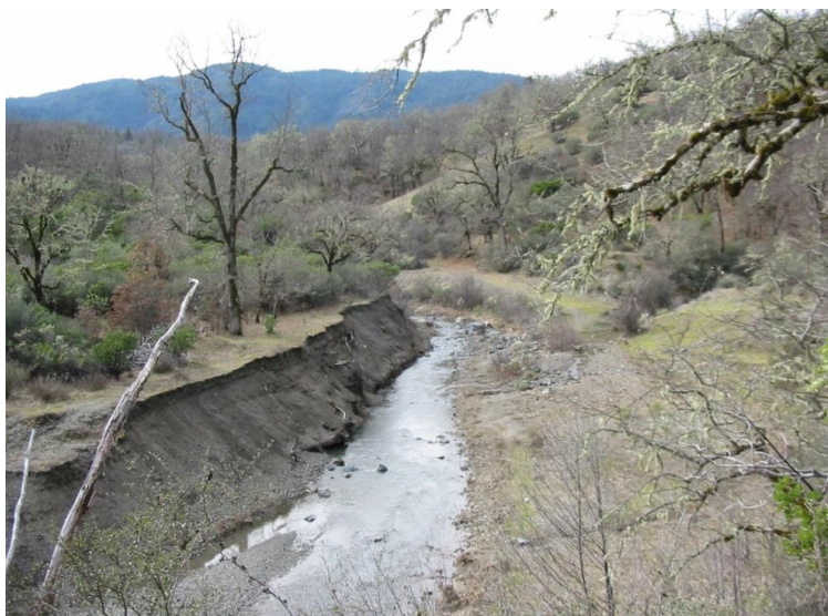
Figure 13. Photograph of the impoundment area of Town Creek near Covelo, California, showing the steep right bank (left of the picture) formed following dam collapse. Photograph was taken on February 6, 2002, standing at the dam site looking upstream.
