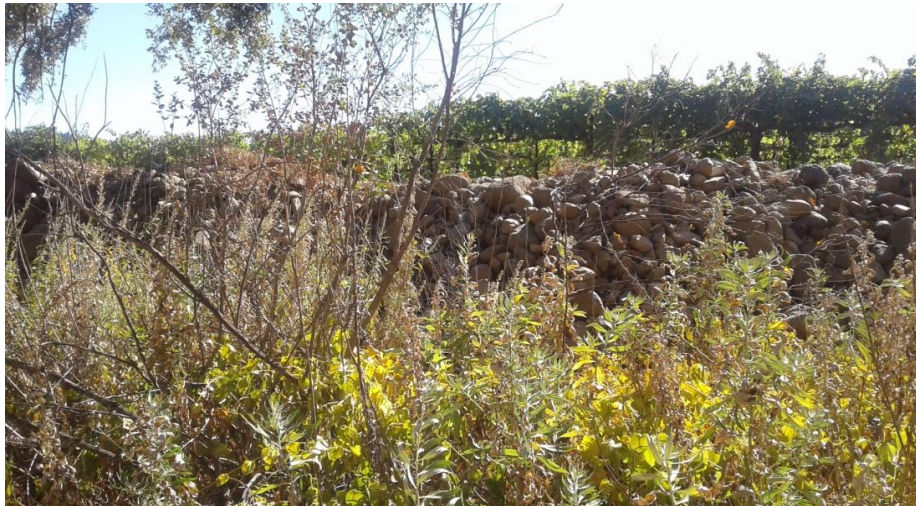
Figure 7. Photograph of gravel/boulder berm placed at the right bank of York Creek near the Napa River confluence. Photograph was taken on September 26, 2017.
