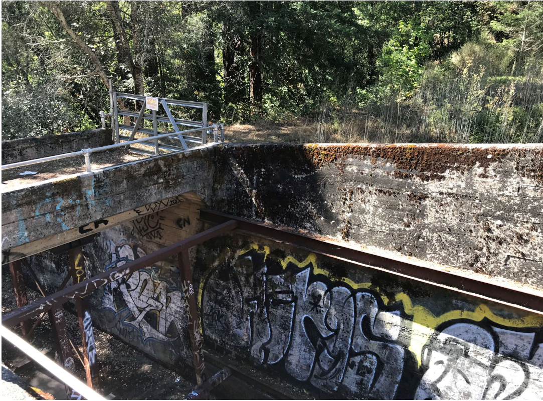
Figure 1-5: The Existing Condition of the Top of Upper York Creek Dam and Spillway with the Access Bridge Shown (Date: 10/9/18)
