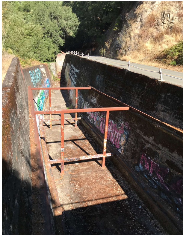
Figure 2-1: Existing Spillway and Spring Mountain Road
