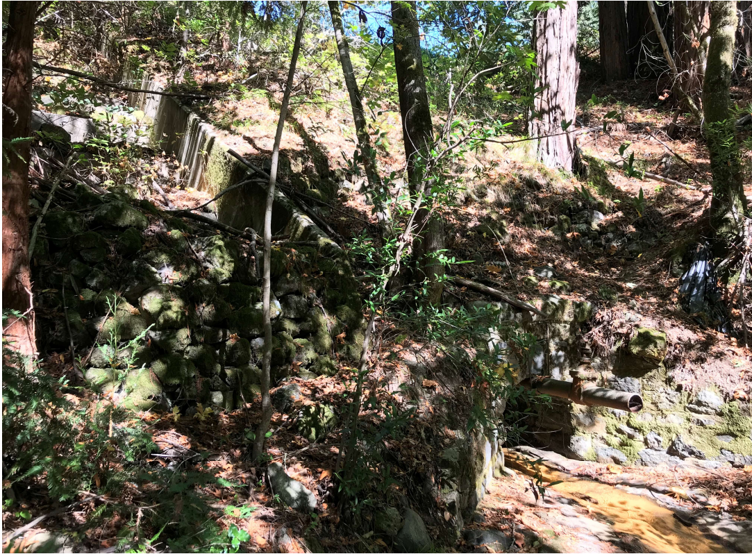
Figure 1-4: Downslope Side of the Upper York Creek Dam Showing the Outlet at the Base of the Dam (Date: 10/9/18)
