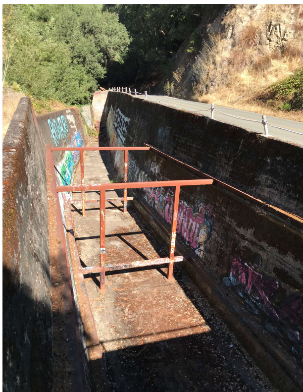
Figure 2-1: Existing Spillway and Spring Mountain Road
