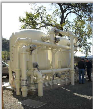
View of new pressure filter train added for redundancy and improved particulate removal
