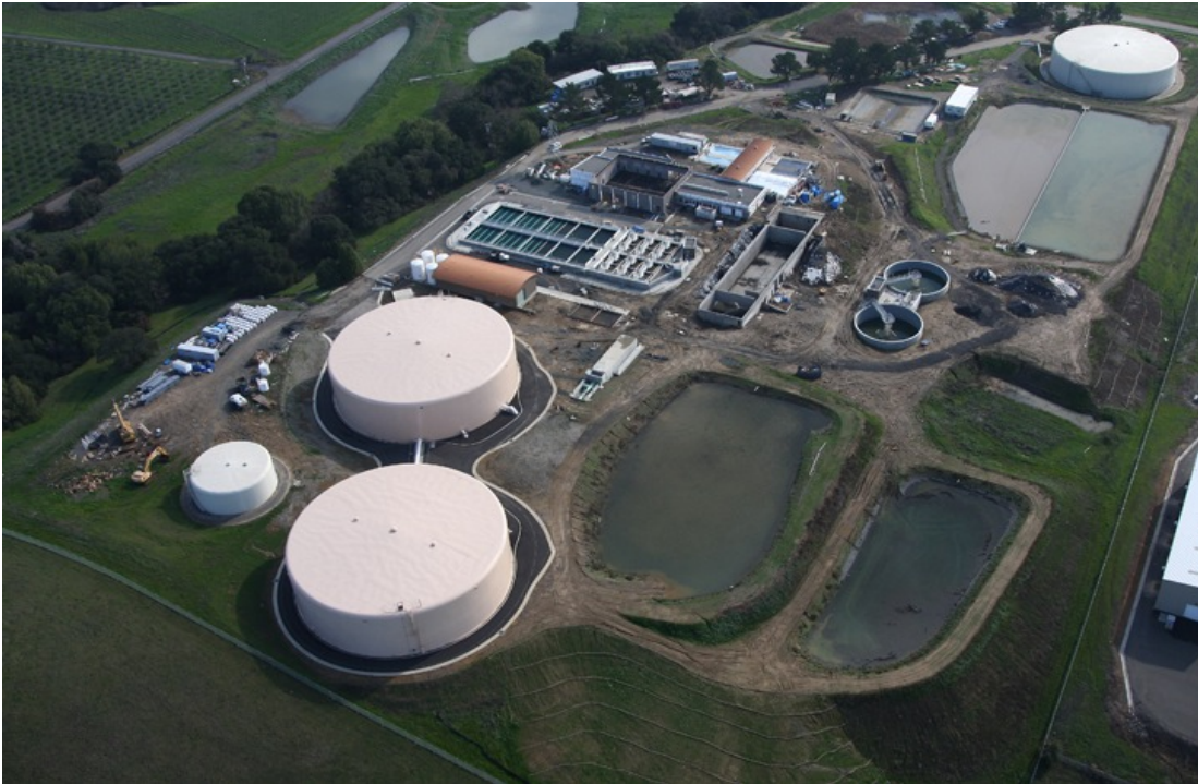
Jamieson Water Treatment Plant aerial view.
