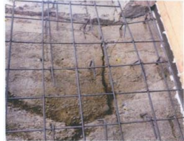
Additional cracking was noted in early May during the temporary repair of Abutment 1.
