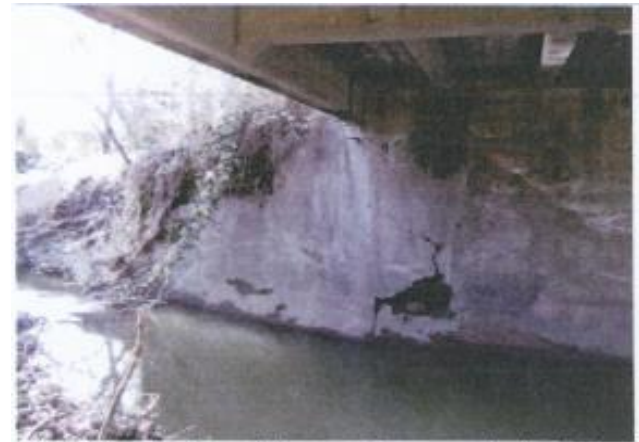
The spall in the face of Abutment 1 was repaired in Spring 2014.
