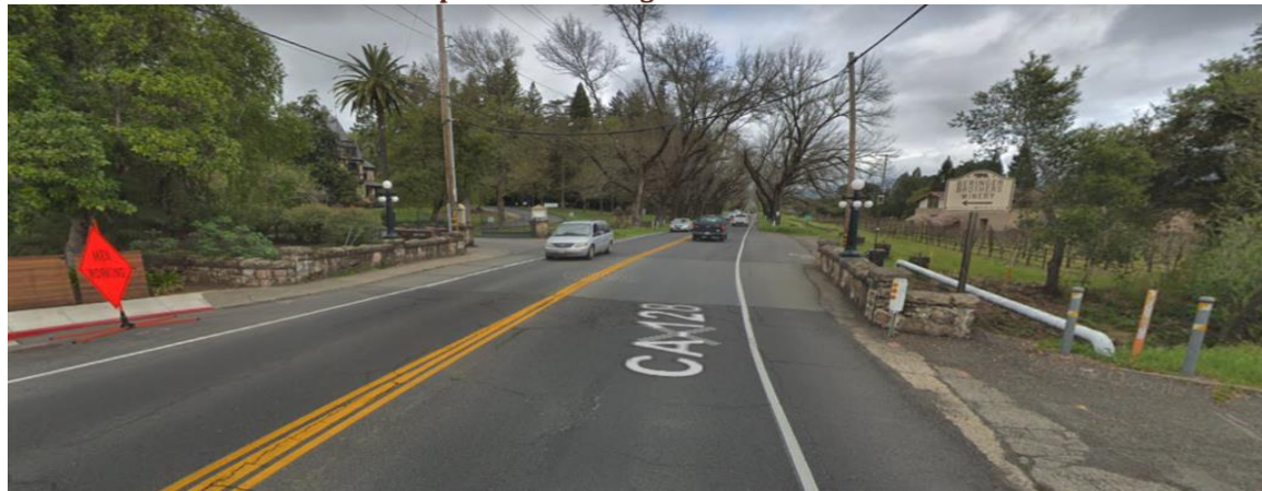
York Creek Bridge
