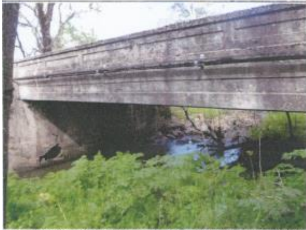
The reinforced concrete Hopper Slough Bridge was built in 1921
