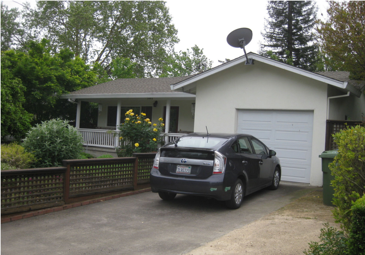
EXISTING RESIDENCE - FRONT/GARAGE ELEVATION
