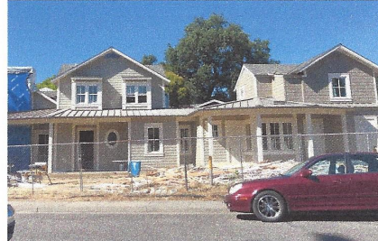
1401 Allyn Ave. – In Progress
