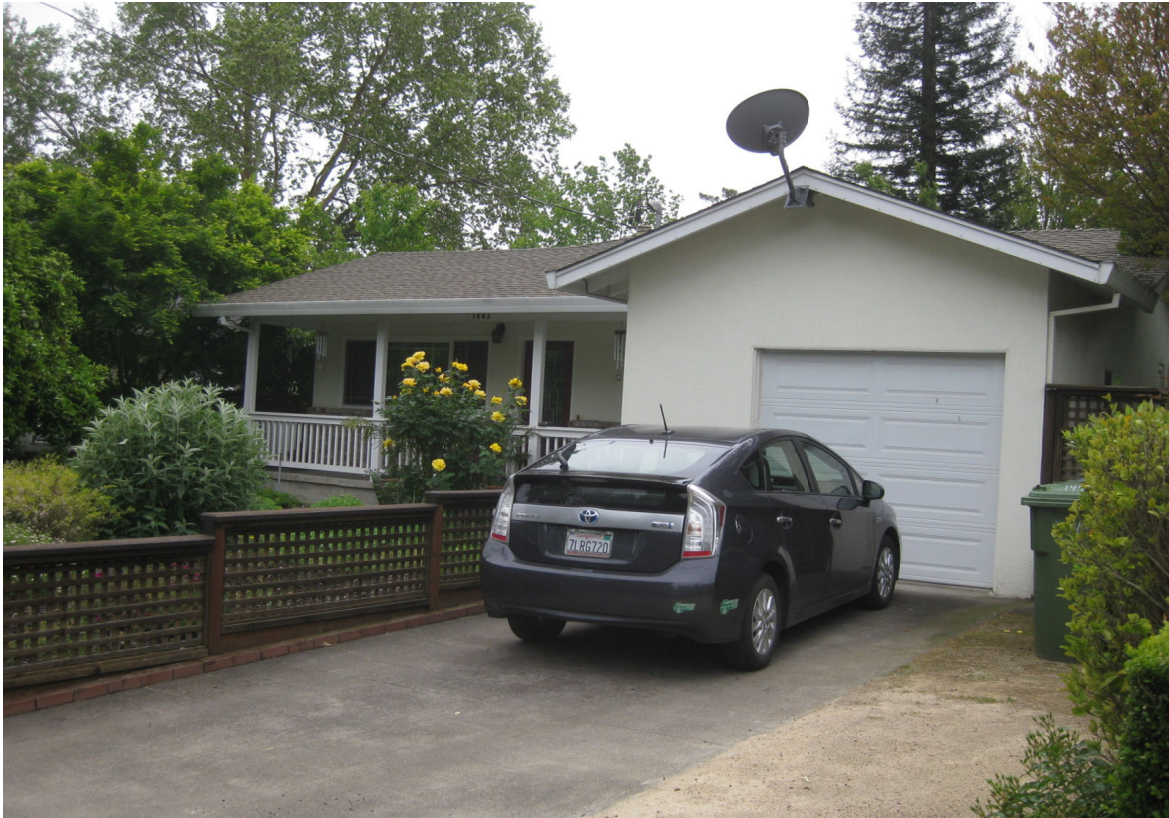
EXISTING RESIDENCE - FRONT/GARAGE ELEVATION
