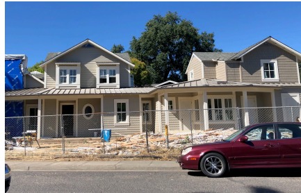
1401 Allyn Ave. – In Progress
