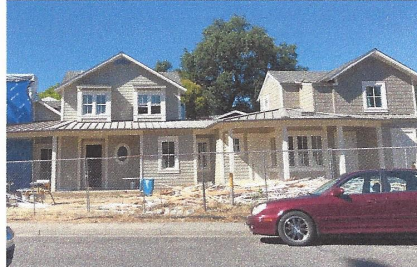
1401 Allyn Ave. – In Progress
