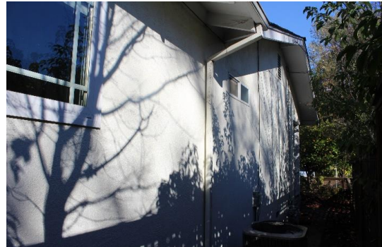
Photograph 5: East elevation, camera facing west, November 16, 2018.
