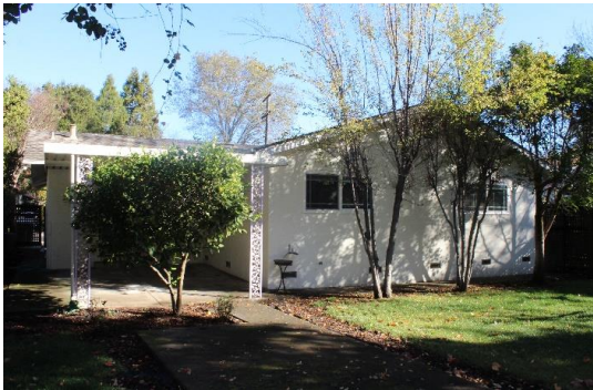
Photograph 6: South elevation, camera facing northeast, November 16, 2018.
