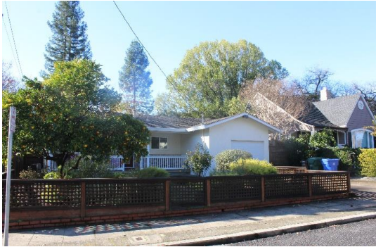
Photograph 2: North elevation, camera facing west, November 16, 2018.
