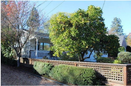
Photograph 4: North and east elevations, camera facing west, November 16, 2018.
