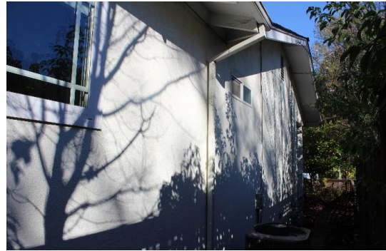
Photograph 5: East elevation, camera facing west, November 16, 2018.
