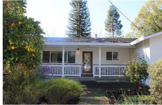
Photograph 3: Detail, north elevation, front door, camera facing southwest, November 16, 2018.
