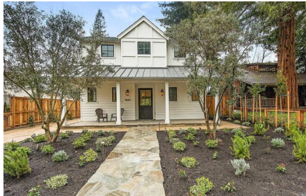
1645 Vineyard Ave – Completed 2018
