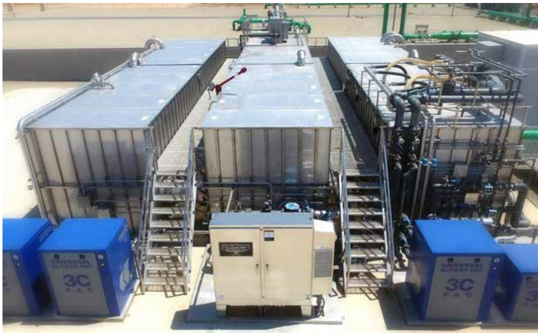
Figure 4-3: Example of Pre-Engineered, Packaged MBR Treatment Plant (Cloacina, 2019)
