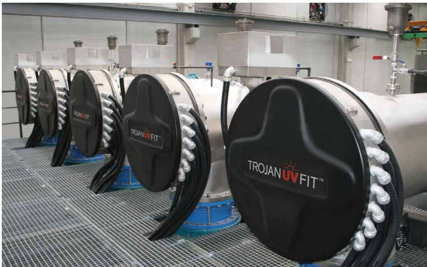
WASTEWATER DISINFECTION FILTERED IN-PIPE TREATMENT
