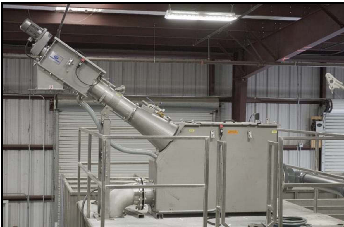
Example Screen Installation
