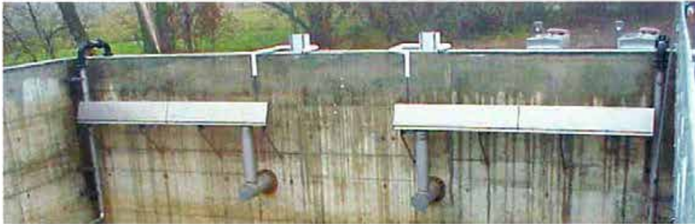
Dual stainless steel fixed air-sealed decanters
