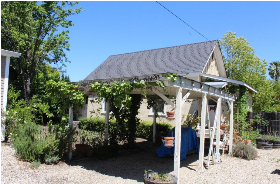
Photograph 2: 1420 Allyn Avenue, southwest and southeast elevations, camera facing northeast, May 10, 2021.
