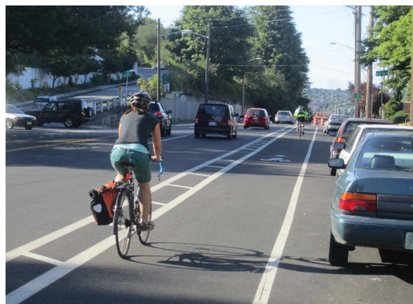
Figure SH.8. Buffered bike lane in Seattle, WA
