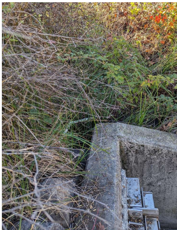
Levee Photo 10: Southwest corner of levee culvert outfall structure. Rock moved for irrigation piping; no scour observed.
