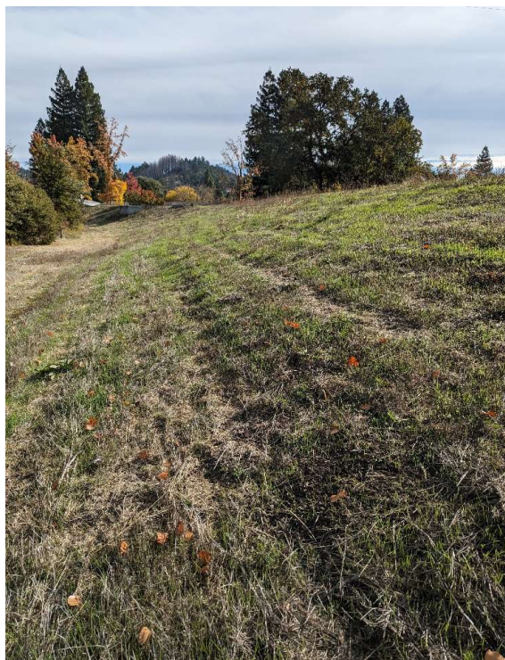
Levee Photo 1: Waterside levee slope recently mowed with adequate vegetation setback.
