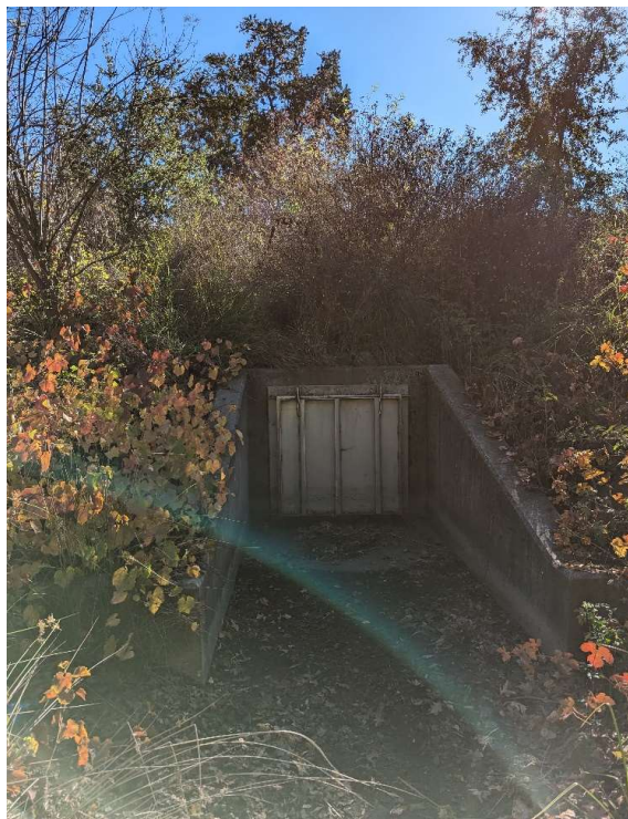
Levee Photo 9: Levee culvert outfall structure. Vegetation maintained to allow flap gate operation and free discharge.
