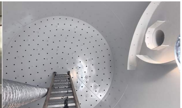
Prep and Epoxy Coatings of Steel Vertical Filter
