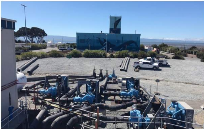
Bypass and Coating of Effluent Discharge Channel
