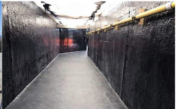
Bypass and Coating of Effluent Discharge Channel
