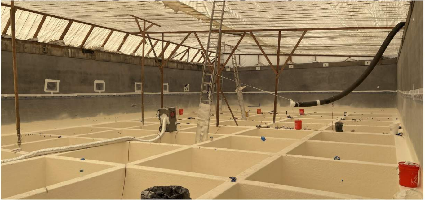
ENDURA-FLEX 1988 Polyurathane Coating 250mil on Concrete
