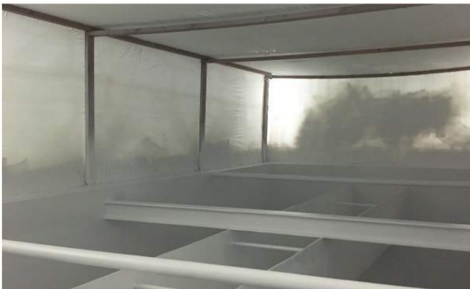
Containment and Epoxy Coating of Microfloc Filter
