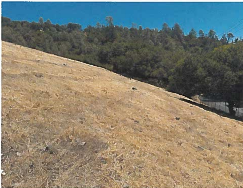
Photo 2: View of the downstream slope observed from near the right groin.
