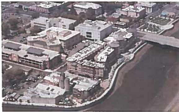
Completed Project from Above
