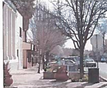
Oak Street - Angle parking prior to sidewalk widening
