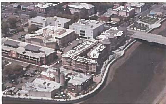
Completed Project from Above
